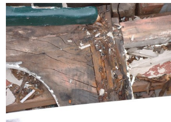
One of her knees and rotten deck beams
