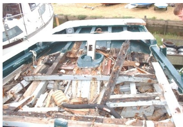
The deck and deck beams have been removed exposing her counter
