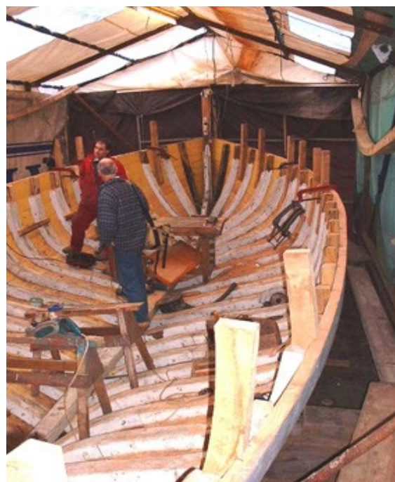
The stanchions are now going in including the stanchions for the barrel windlass.
