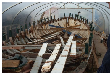
Seen here the deck has been removed and her hull has been braced
