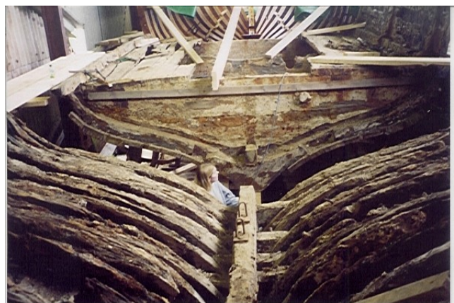
The old frames and wet well.
