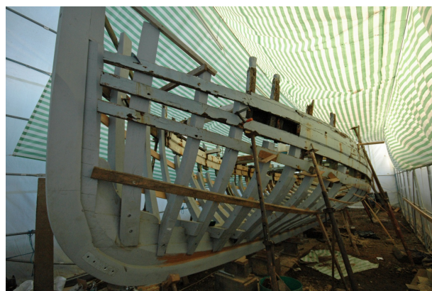
Keel, stem, apron and knee. Original planking and battens preserve the original shape.
