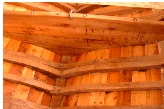
Re creating the 'wet well'
